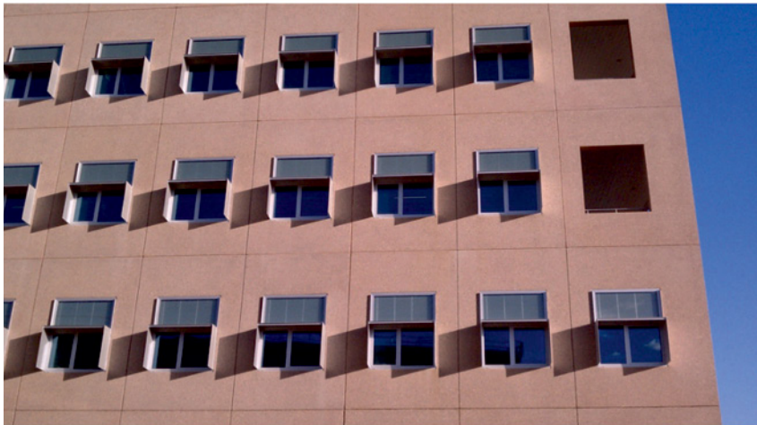
Figure 7.3 Intelligent façade which incorporates architectural innovations that reconfigure the subsystems by integrating several components and functions. In this picture, the fenestration for the National Renewable Energy Laboratory (NREL) Research Support Facility (RSF) which was designed to provide excellent daylighting while controlling glare and solar thermal gain through the use of shading devices, recessed windows, and electrochromic glass.
