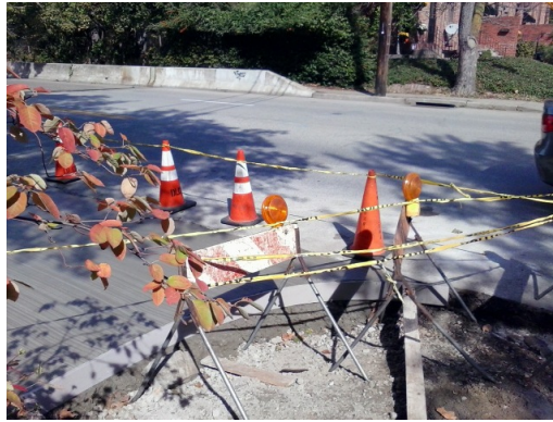
Figure 7.1 A wooden spline used to create a smooth, curved border for a paved area (Shadyside, Pittsburgh, October 2014).
