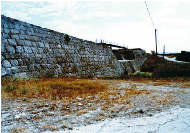
Fig. 29. The GROTTICELLI masonry weir on the Gela River in Sicily, built in 1563 and designed by Architect Carlo Cadorna (photo by C. Gambino)
