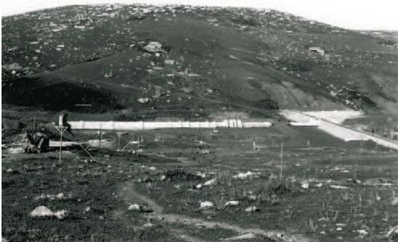
Fig. 116. The TRINITA' embankment dam under construction on the Delia River in Sicily in 1955. The outlet culvert crosses the dam foundation; one can note the reliefs at the extrados in order to improve contact of the concrete with the embankment core material [6] (photo by R. Jappelli, 1955)
