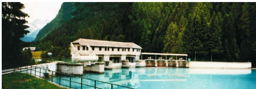
Fig. 50. The small BRUSSON dam in Val d'Aosta, Italy (1928) (photo by S. Di Maio, 1996)
