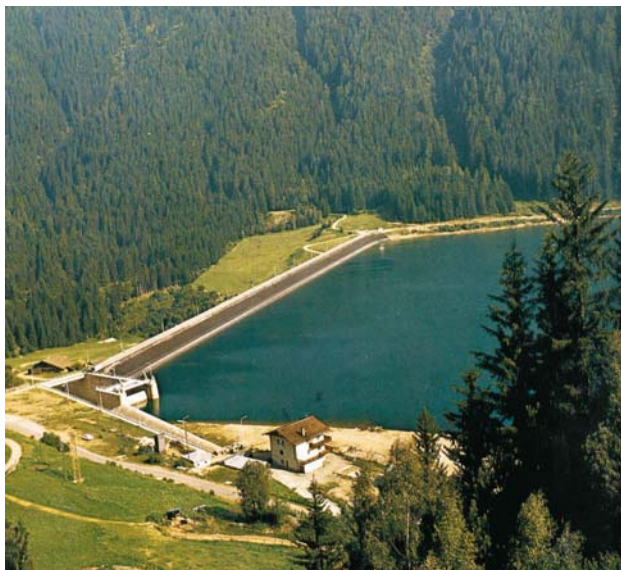
Fig. 36. The ZOCCOLO dam and reservoir from the left bank with the spillway and the guardhouse in the foreground [63]
