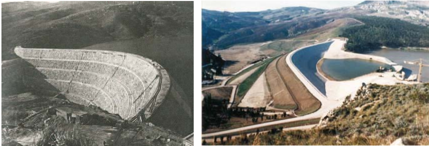
Fig. 40. A. The old DISUERI dry masonry dam (1948); B. The new DISUERI embankment dam (1994) with higher normal water level elevation
