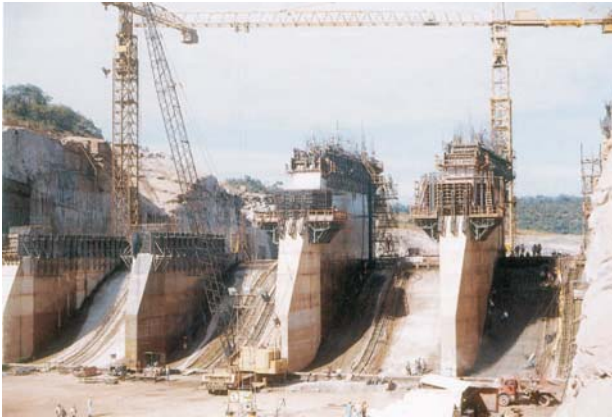
Fig. 47. The spillway of a large Brazilian dam under construction
