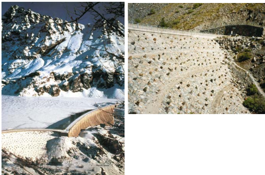
Fig. 49. The CIGNANA dam (1928) in Val d'Aosta, Italy, with a close-up view of the handplaced masonry facing on the downstream slope
