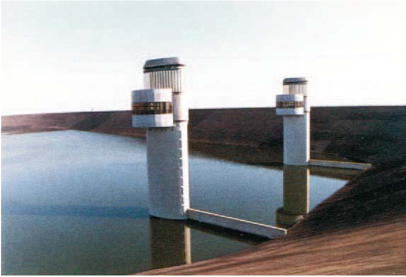
Fig. 70. The upper reservoir of the ANAPO pumped storage hydroelectric plant with its intake towers
