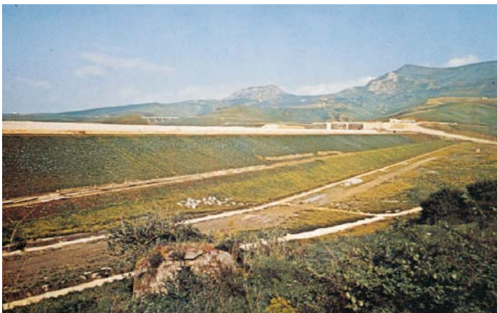
Fig. 57. The GARCIA embankment dam on the Belice Destro River, Palermo
