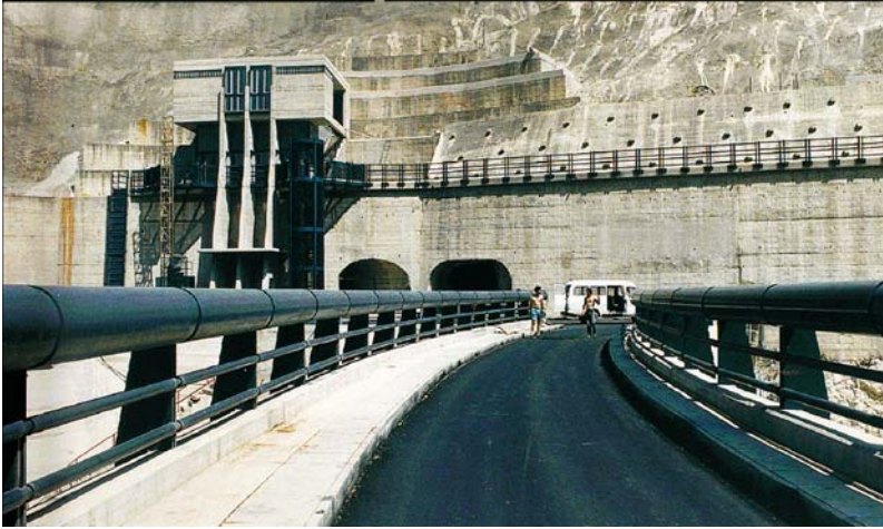
Fig. 53. The guardhouse with the station for operating the outlet valves and for the acquisition and digest of instrument results installed at the ROSAMARINA dam on the San Leonardo River near Palermo, Italy (photo by C. Gambino, 2002)
