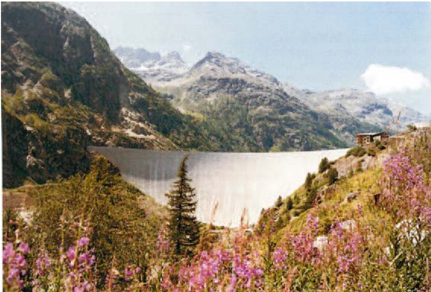
Fig. 9. The PLACE MOULIN is an arch gravity dam on the Buthier River in Val d'Aosta, Italy [64]
