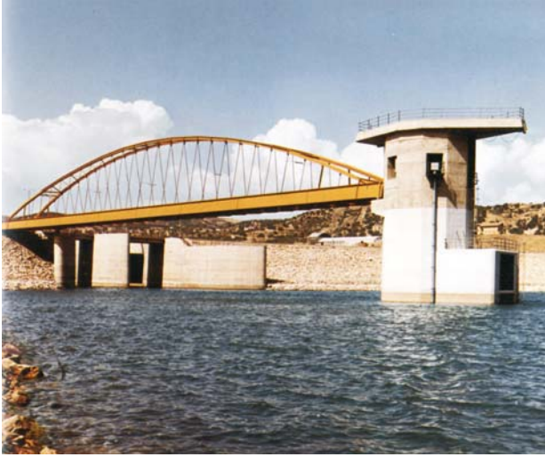
Fig. 51. The metallic footbridge (design by F. De Miranda) to access the intake tower of the VILLAROSA reservoir on the Morello River near Enna, Sicily [6]
