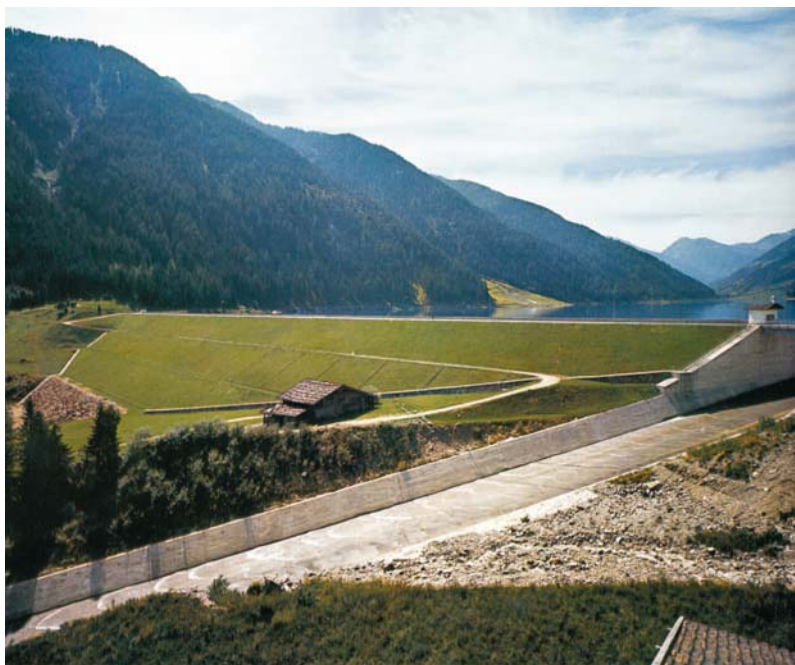
Fig. 79. The ZOCCOLO embankment dam in Val d'Ultimo, near Trento, Italy, from downstream; the spillway open channel in the foreground [63]
