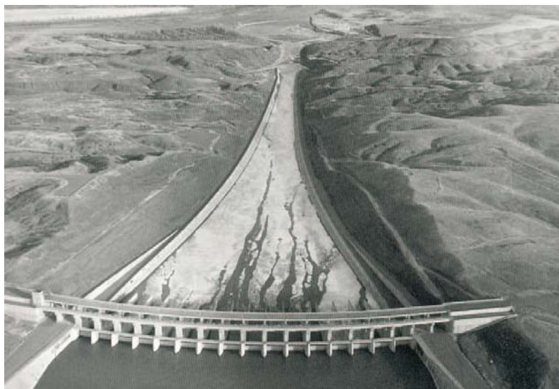
Fig. 93. The spillway of the FORT PECK dam from upstream [136]
