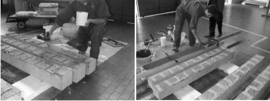
Fig. 1. Restoration phase, anti-corrosion treatment of the irons (a) and volume reconstruction (b)
