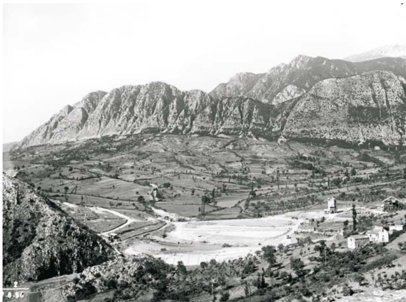
Fig. 76. The CASTELSANVINCENTO embankment dam near Isernia, Italy, under construction in 1956; the Mainarde chain of mountains rises in the background (photo by G. Chiolini)
