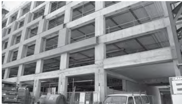
FIGURE 13.6 Concrete moment framed building.
