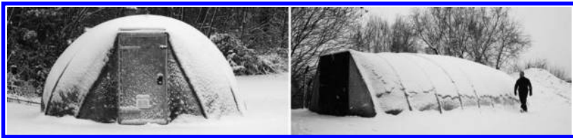
FIGURE 11.14 Concrete canvas structure in cold climate. (From London Royal College of Art, Concrete Canvas , London, United Kingdom, Accessed on February 6, 2015, http://www.rca.ac.uk/research-innovation/innovation/innovationrca-start-up-and-fellowship-projects/concrete-canvas/ , 2015.)
