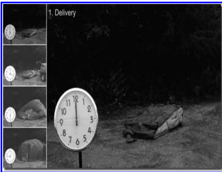
FIGURE 11.12 Concrete canvas as delivered to the site. (From London Royal College of Art, Concrete Canvas , London, United Kingdom, Accessed on February 6, 2015, http://www.rca.ac.uk/research-innovation/innovation/innovationrca-start-up-and-fellowship-projects/concrete-canvas/ , 2015.)
