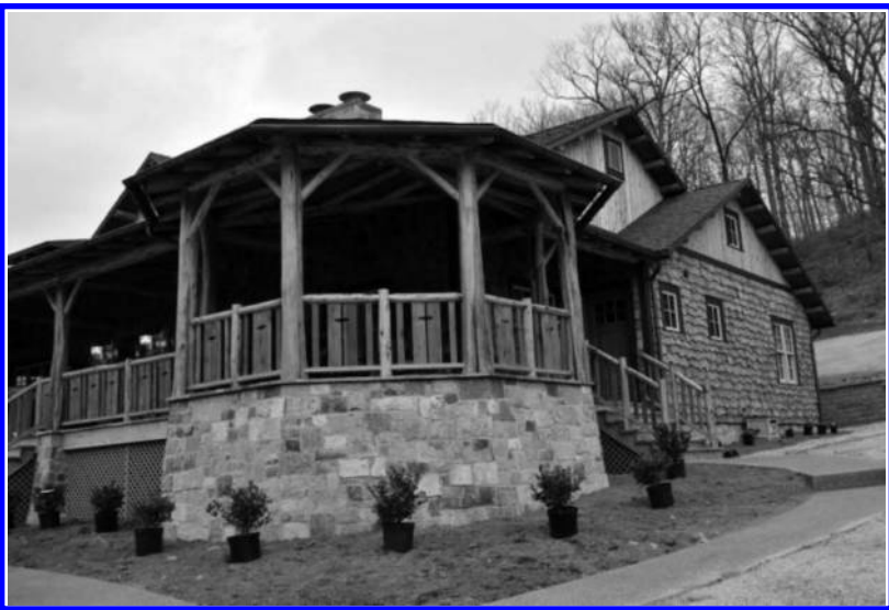
FIGURE F.4 HomeWaters main building front deck side view. (Courtesy of Samuel Seltzer.)
