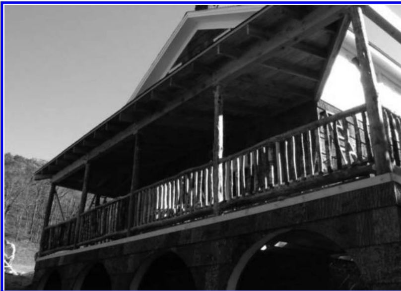
FIGURE F.2 HomeWaters main building upper deck. (Courtesy of Samuel Seltzer.)
