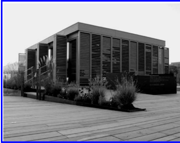
FIGURE 13.11 Building retrofitted with louvered photovoltaic panels. (From Das Haus, Innovation in Renewables and Energy Efficiency , Federal Ministry of Economics and Technology, Federal Ministry of Transport, Building and Development, Berlin, Germany, Accessed on December 19, 2014, http://www.inefficiency-fromgermany.info/ENEFF/Redaktion/EN/Downloads/Publikationen/das_haus_%20innovation_in_renewables_and_energy_efficiency.pdf?__blob=publicationFile&v=5 , 2011.)
