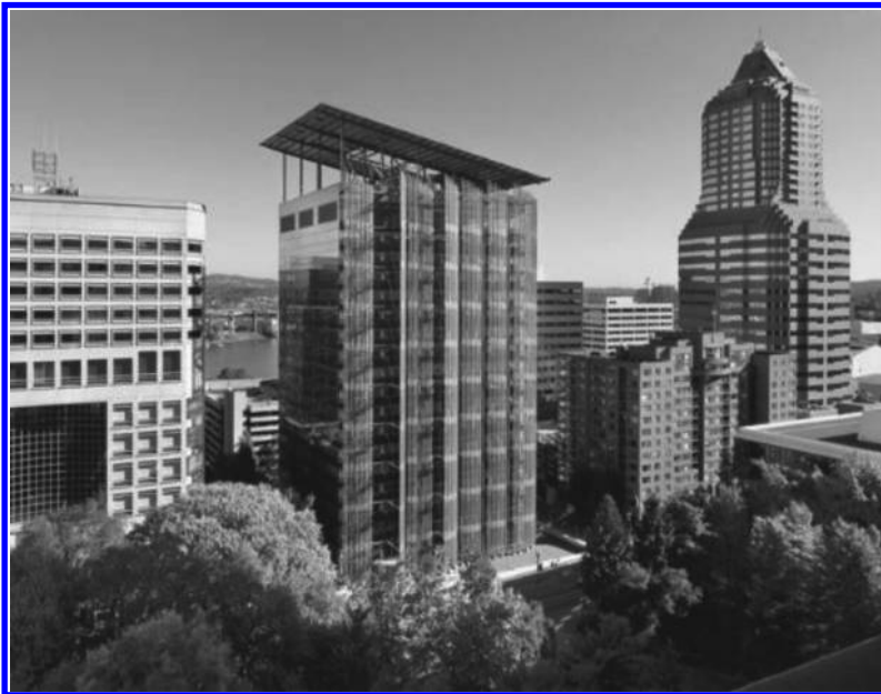
FIGURE 10.1 Green building skin on the Portland federal building. (Government Services Administration, Edith Green–Wendell Wyatt Modernization Project—Portland, Oregon Federal Building , Portland, Oregon, Accessed on February 5, 2015, http://gsa.gov/portal/content/252613 , 2014.)
