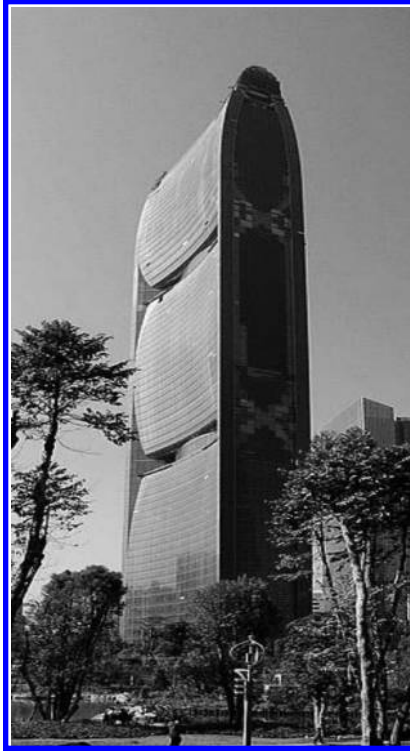
FIGURE 13.7 Chinese high-rise structure with embedded wind turbines. (Open source photograph.)
