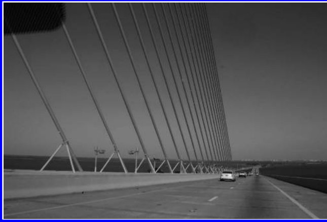
FIGURE 11.10 Sunshine Skyway Bridge in Tampa with 30% fly ash in the concrete mix. (Authors.)
