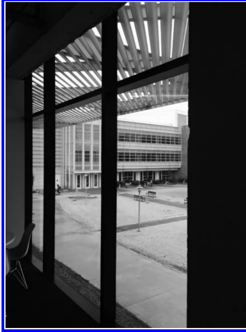
FIGURE 14.2 Study lounge high-performance windows; Mason Building, Georgia Institute of Technology, Atlanta, Georgia. (Courtesy of Daniel Castro-Lacouture.)
