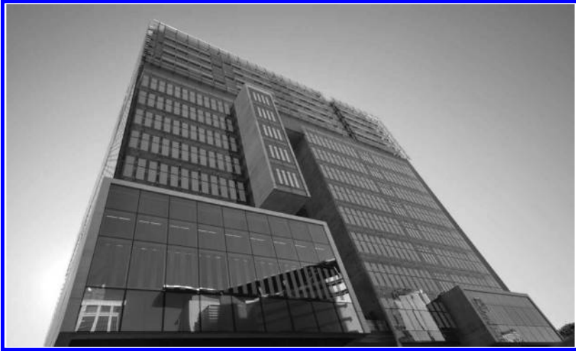
FIGURE 13.3 Photovoltaic skin on the Brisbane Supreme and District Court Building. (From Queensland Government, Courts and Tribunals , Brisbane, Australia, Accessed on February 17, 2015, http://www.justice.qld.gov.au/justice-services/courts-and-tribunals/our-courthouses/new-brisbane-supreme-and-district-court , 2015.)
