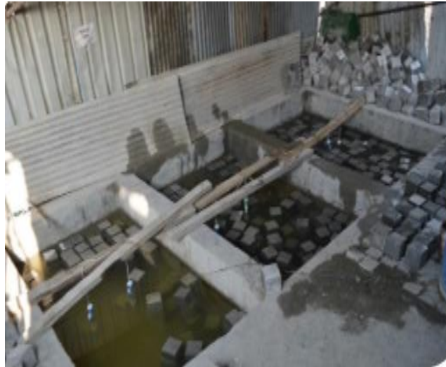
Figure 3.8: (b) Curing of Concrete Cubes
