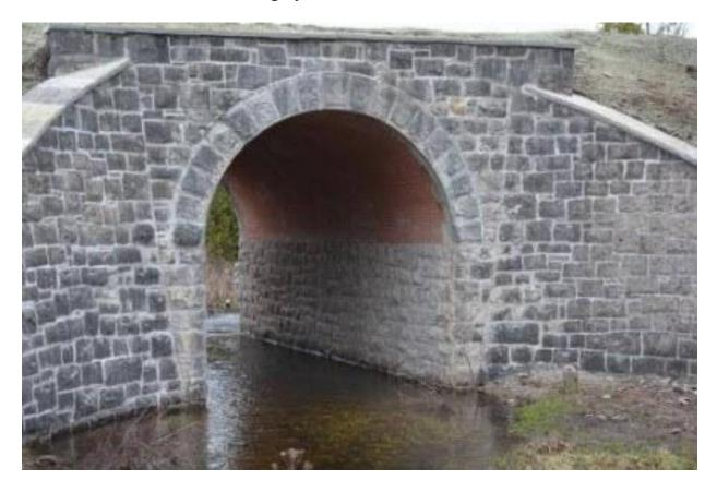
The advantages of using arch culverts over traditional box culverts and pipe culverts are as follows:
