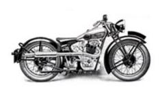
1933 The Bullet Arrives-In 1931 a four-valve, single-cylinder was introduced, and christened 'Bullet' in 1932. It had an inclined engine and an exposed valve gear.
