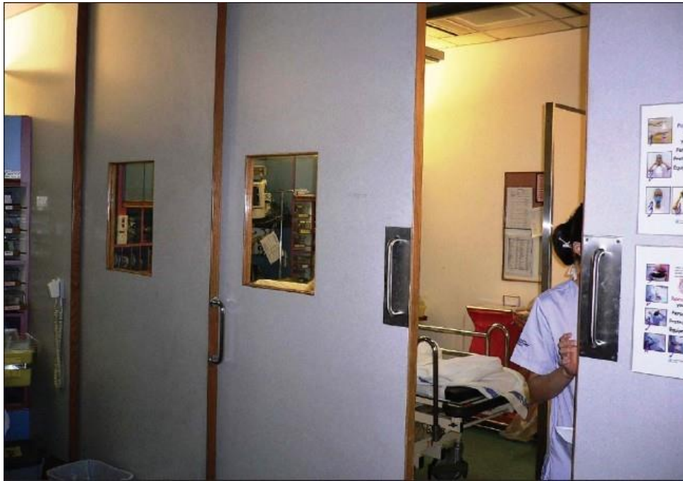
Figure 4 Negative pressure ventilation end cubicle in the resuscitation area with lead X-ray proof door partitions
