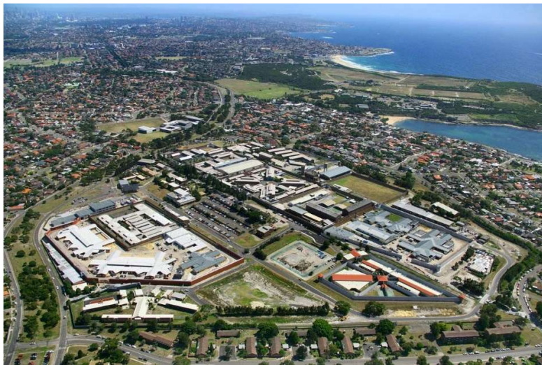
Figure 69: Long Bay Prison's Aerial View.
