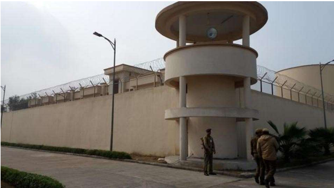
Figure 55: Watch Tower, High Perimeter wall with barbed wires as Main security of Prison.
