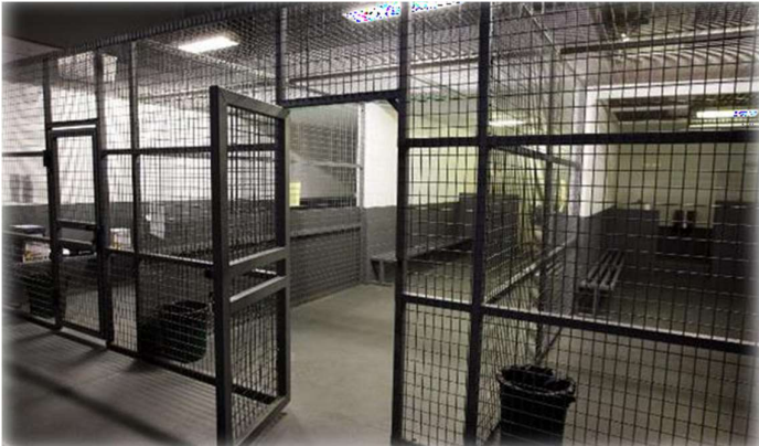
Figure 73: Inside view of the Long Bay Prison.
