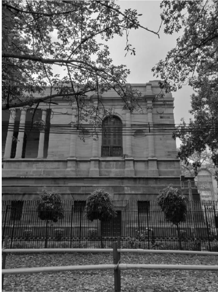
Fig 4.2: National Archives of India Source: Taken by author on site
