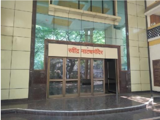
Fig 5.15: Exterior of the building showing the materiality Source: Taken by author
