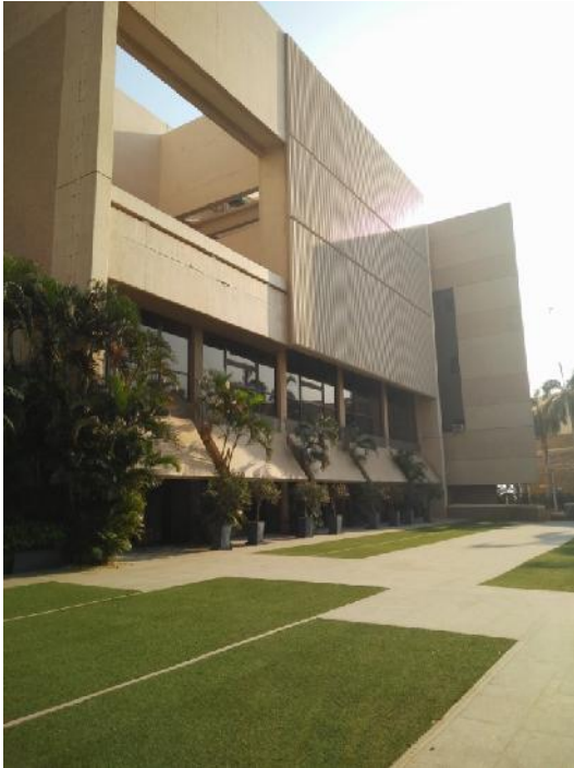
Fig 5.9: Exterior view of the Bhabha Theater Source: Taken by author
