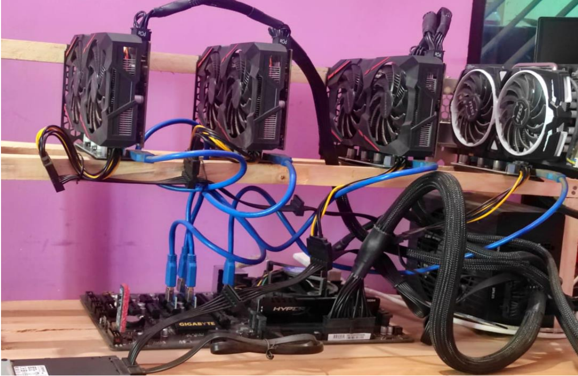
Fig 9. This is a hardware connections of 4XGPU Mining Rig which we have configured.
